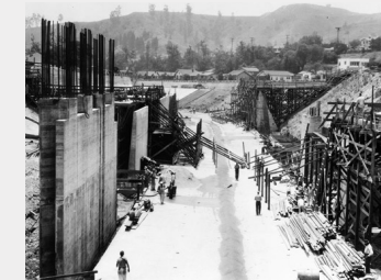
L.A. River is channelized in concrete due to major floods
