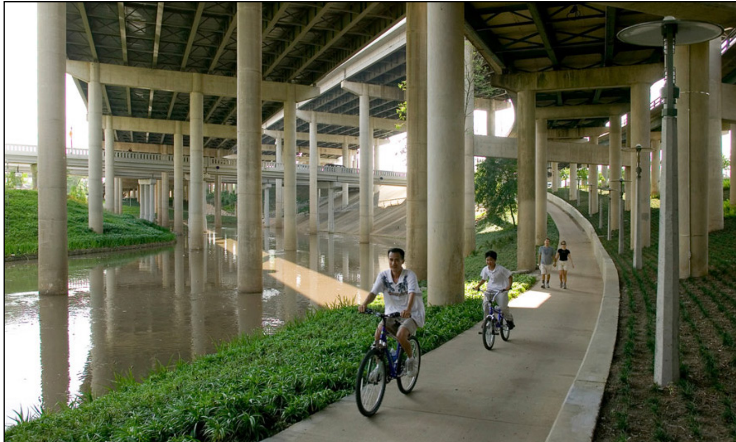
View of the pathway underneath the elevated highways.
